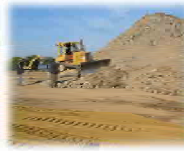
5. Replacing of mixed soil
