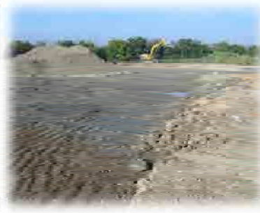
1. Soil removal until clay basement
